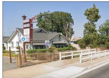
Historic character buildings.
