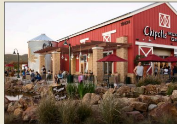
Agricultural-inspired building with outdoor seating and water feature.
