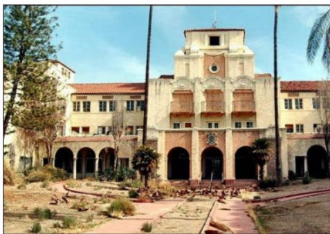
The Norconian hotel is currently vacant and in need of renovation.
