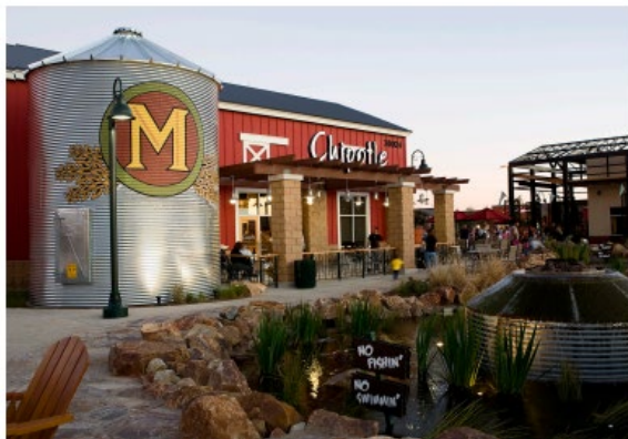
Commercial building with pergola over outdoor dining.
