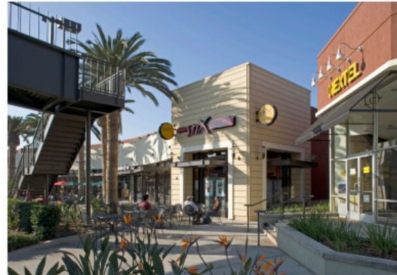
Commercial building with ground floor retail.
