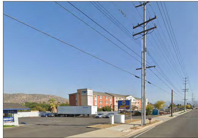
Missing streetscape and parking lots between the street and building.
