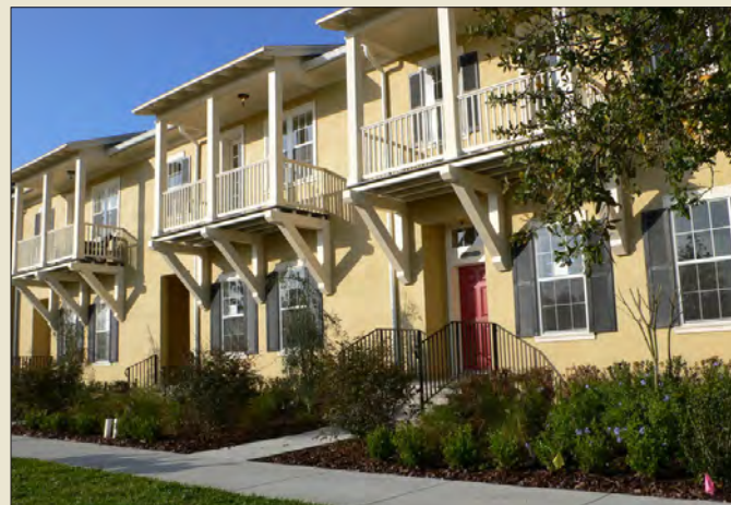
Rowhouses with street-facing entries and upper floor balconies.
