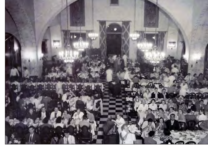
Inspiration for potential future uses – the Norconian Hotel's historic dining room . . .
