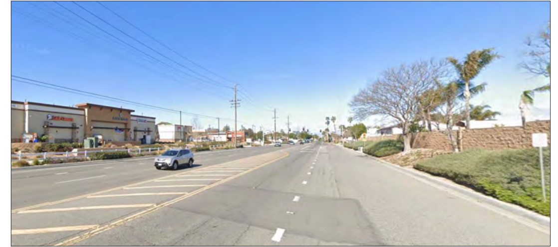
River Road is fronted by the Norco Village shopping center located behind parking lots and a fence-lined trail and single-family residences located behind concrete masonry walls.
