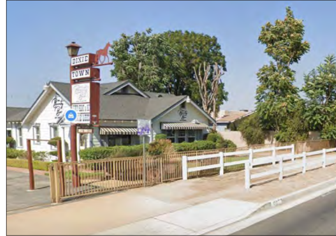
Historic character buildings.
